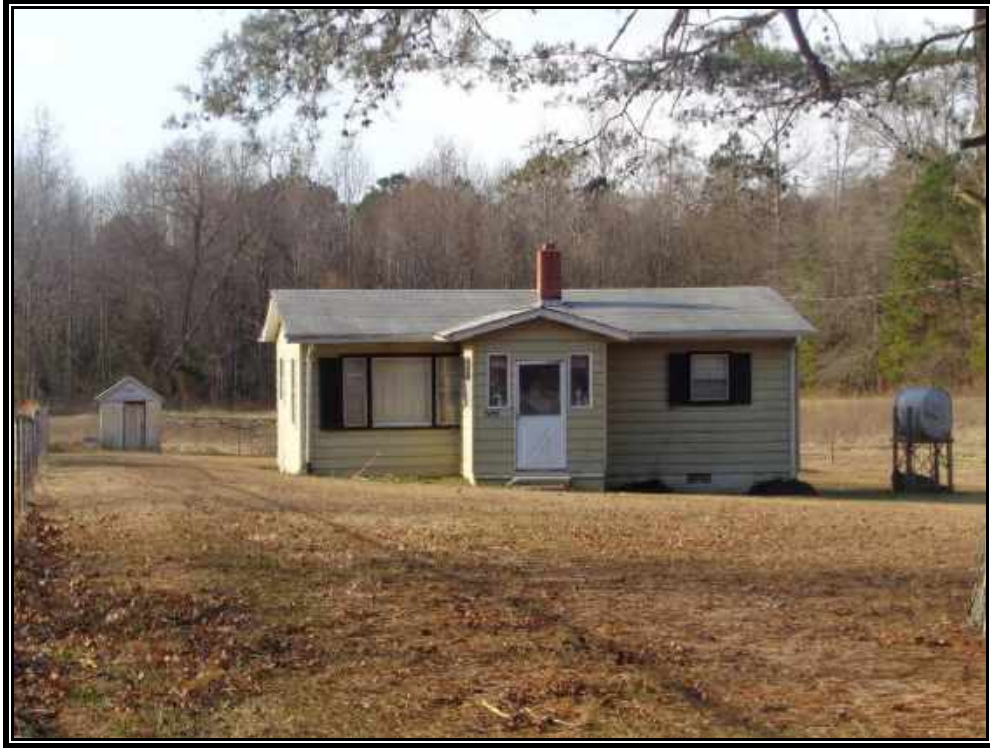
Plate 30. View of Site 090-5091, House, façade, and Shed 1, looking south.
