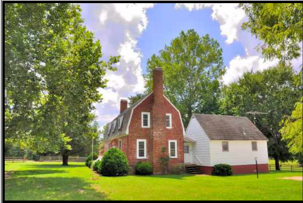
Plate 2. View of Site 090-0012, Main house, side elevation and additions, looking southwest.
