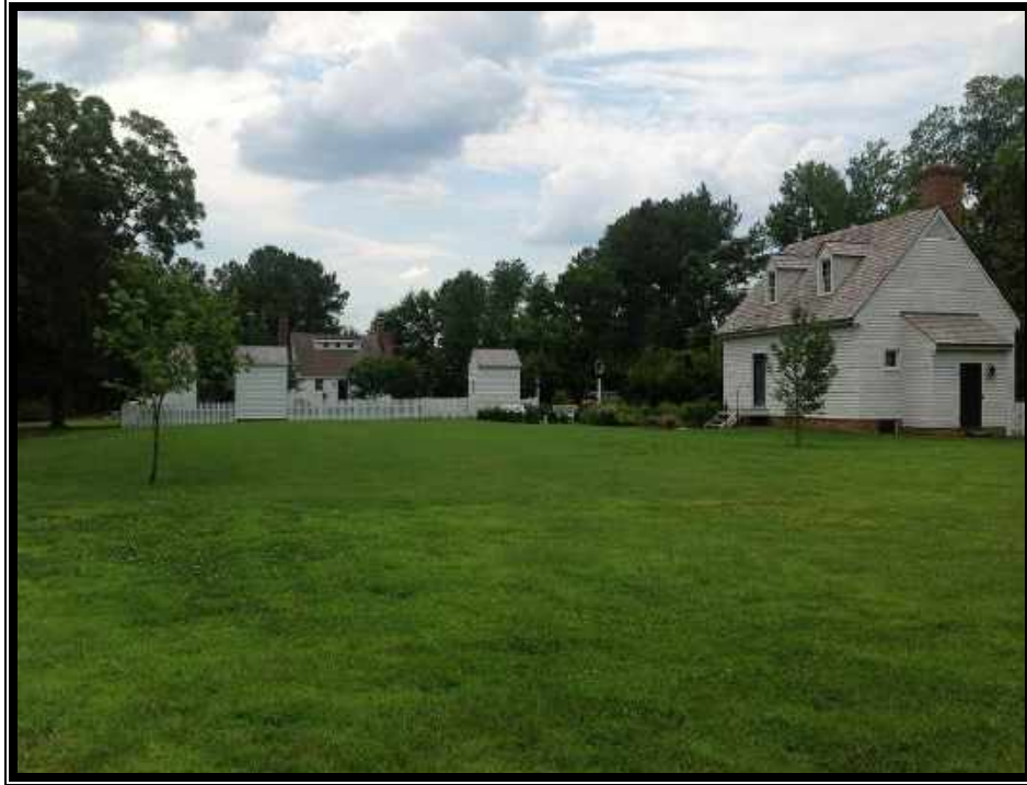
Plate 11. View of Site 090-0036, House, rear elevation; Cottage, façade, side elevation, and addition; and Outbuildings, looking south.
