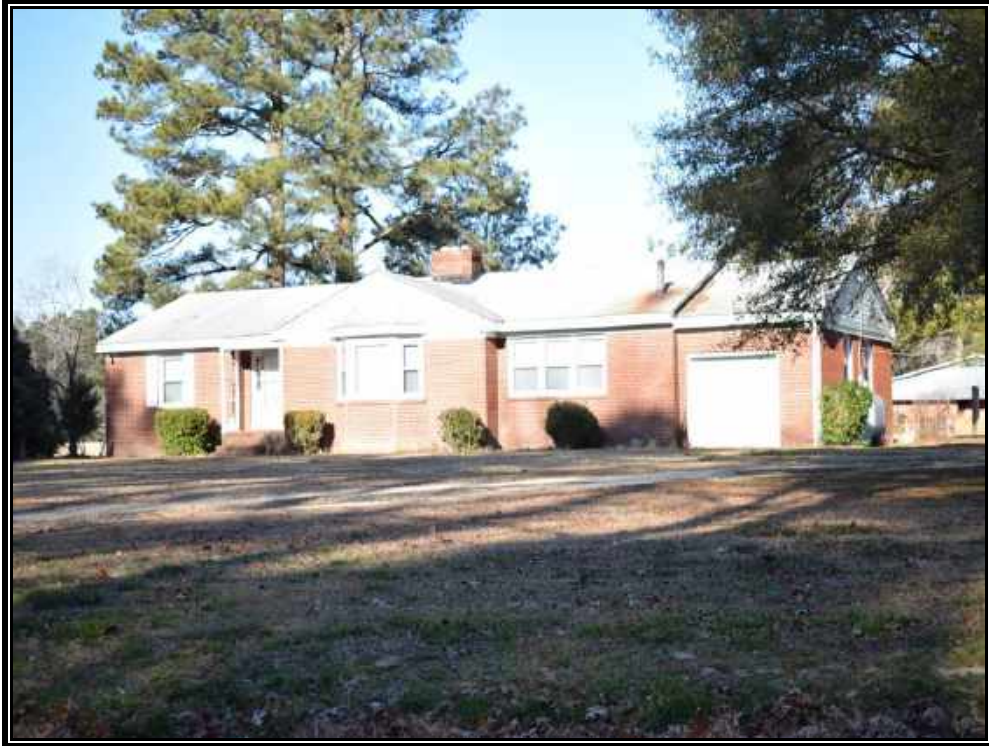
Plate 45. View of Site 090-5095, House, façade, side elevation and addition, looking north.
