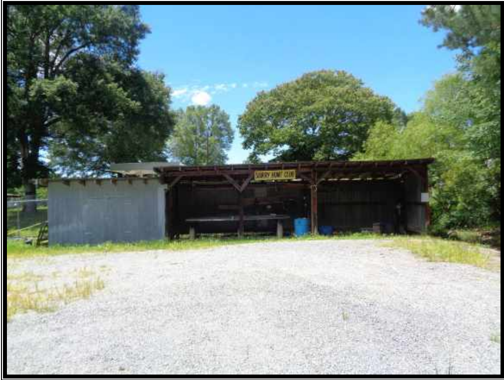
Plate 16. View of Site 090-5070, Pole barn, façade, looking west.
