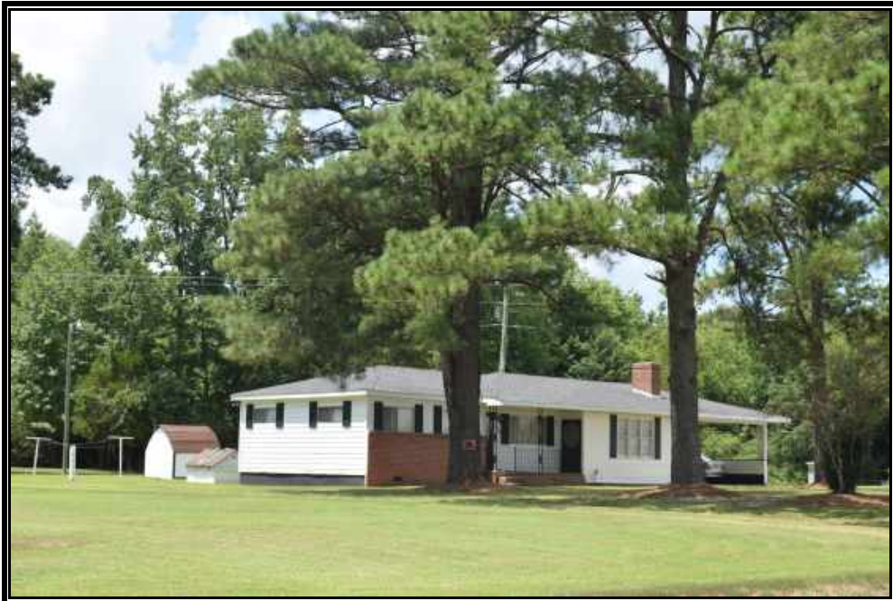
Plate 44. View of Site 090-5141, House, façade, side elevation, and addition, Shed 1, and Well house, looking north.
