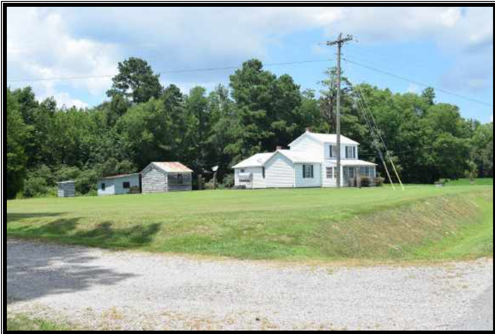
Plate 42. View of Site 090-5140, Secondary dwelling, façade, side elevation, and addition, Sheds 3, 4, and 5, and Well, looking northwest.
