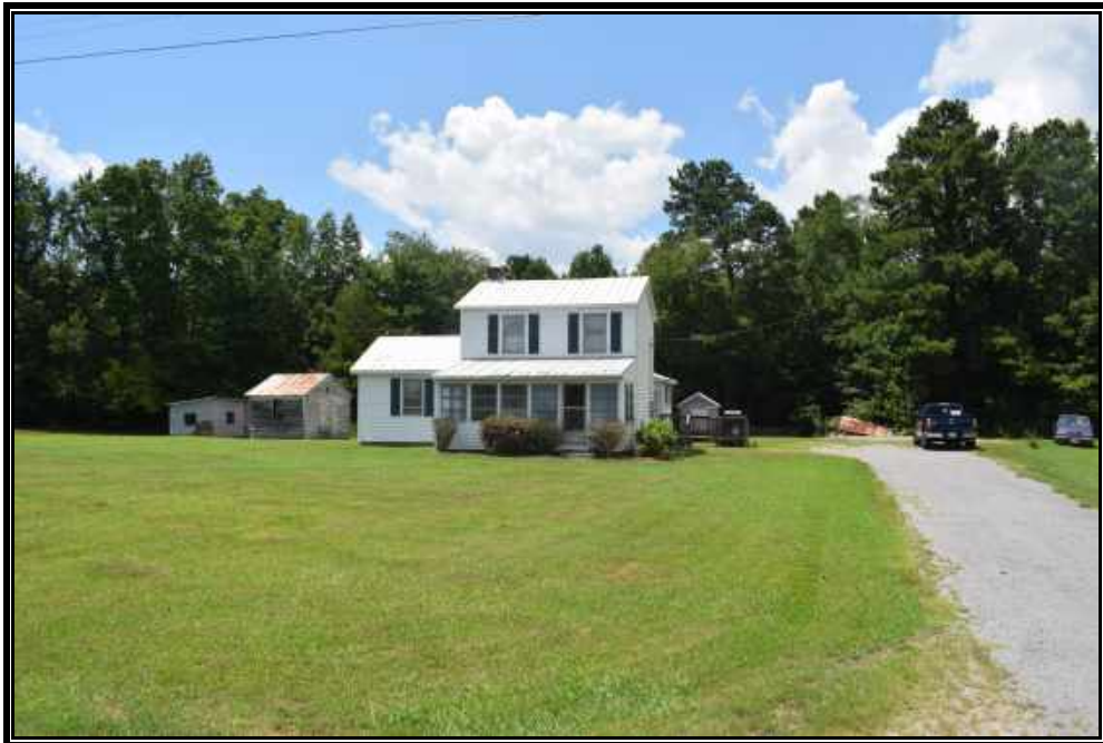
Plate 32. View of Site 090-5140, Secondary dwelling, façade, side elevation and additions, Sheds 2, 3, and 4, and Ruin, looking northwest.
