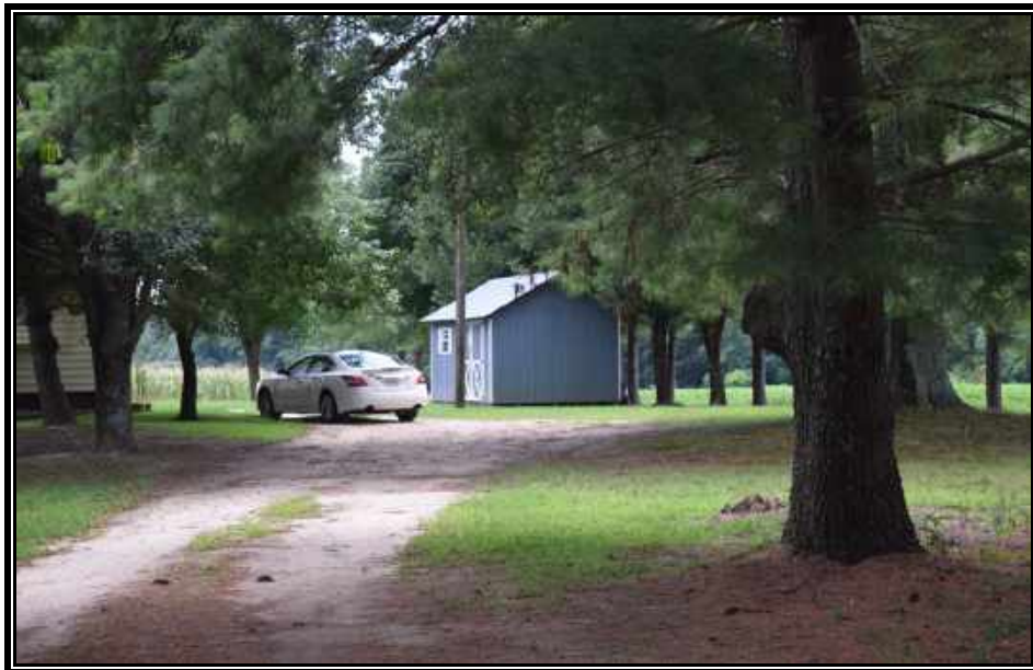
Plate 55. View of Site 090-5144, House, façade, and Shed 1, looking south.
