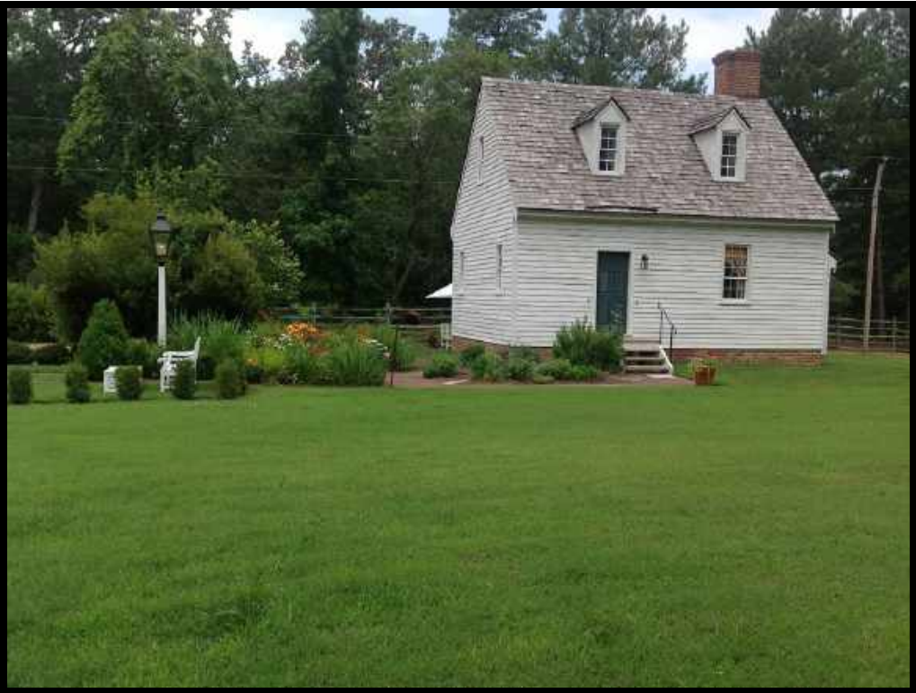
Plate 10. View of Site 090-0036, Cottage, façade and side elevation, looking north.
