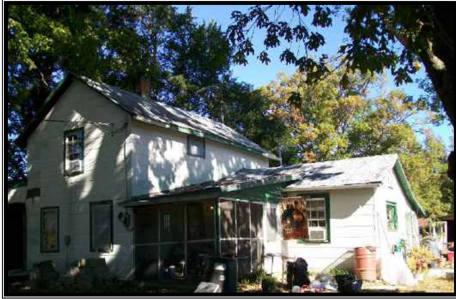
Plate 23. View of Site 090-5074, House, Façade and elevations, looking northwest.
