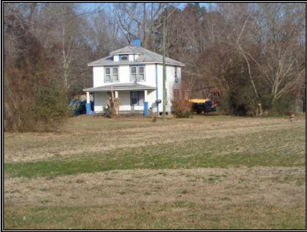
Plate 23. View of Site 090-5089, House, façade, side elevation, and addition, and Shed 1, looking northwest.
