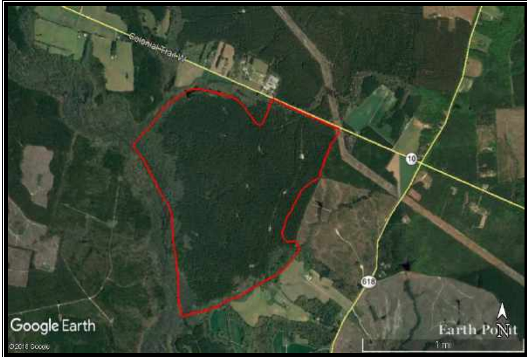
Figure 7. Current (2018) aerial view of project area, from Google Earth.
