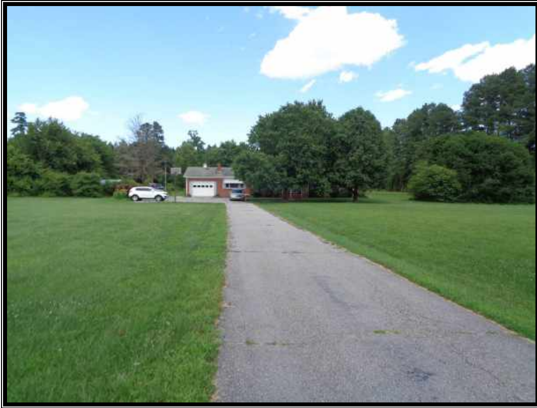
Plate 22. View of Site 090-5073, House, façade, looking north.
