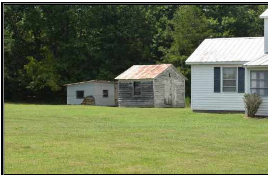
Plate 39. View of Site 090-5140, Secondary dwelling, addition, and Sheds 3 and 4, looking northwest.
