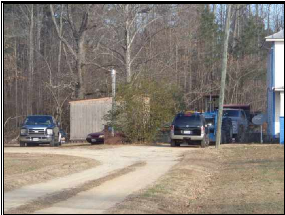
Plate 24. View of Site 090-5089, Shed 1, façade and side elevation, looking north.
