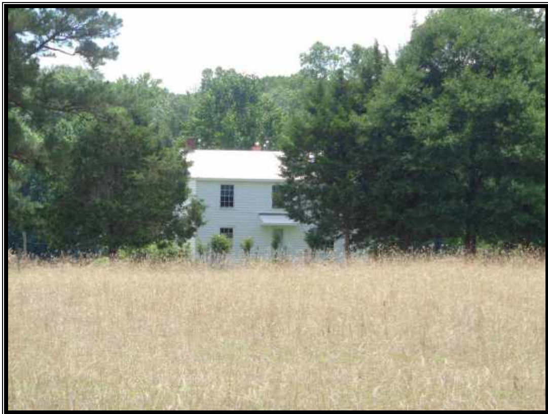
Plate 3. View of Site 090-5075, House, façade, looking south.
