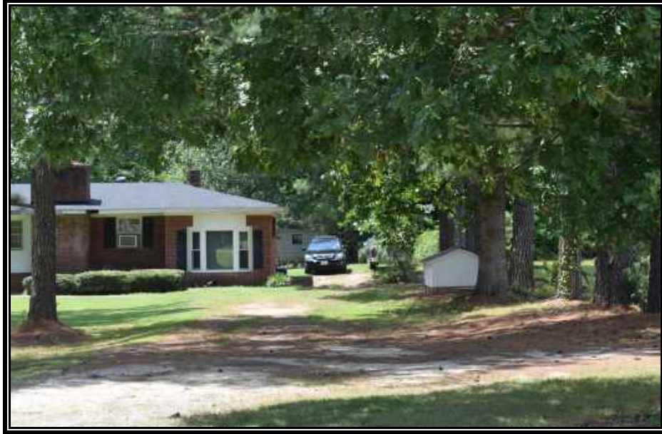
Plate 51. View of Site 090-5143, House, façade and side elevation, Shed, Well house, and Well, looking west.
