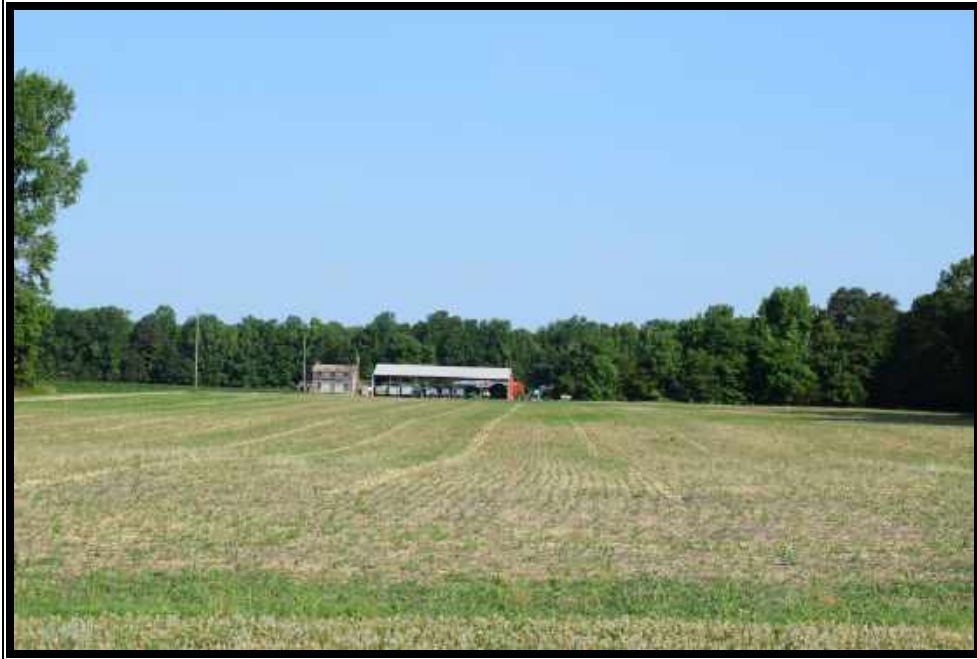
Plate 29. View of Site 090-5140, House, façade and side elevation, and Pole Barns 1 and 2, looking northwest.
