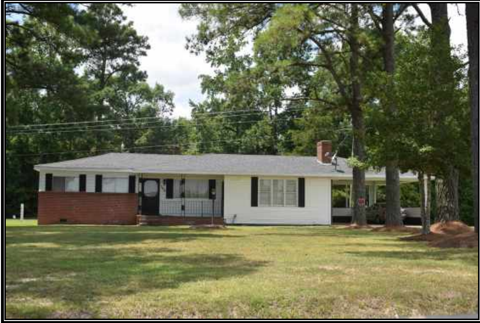
Plate 43. View of Site 090-5141, House, façade and additions, looking west.
