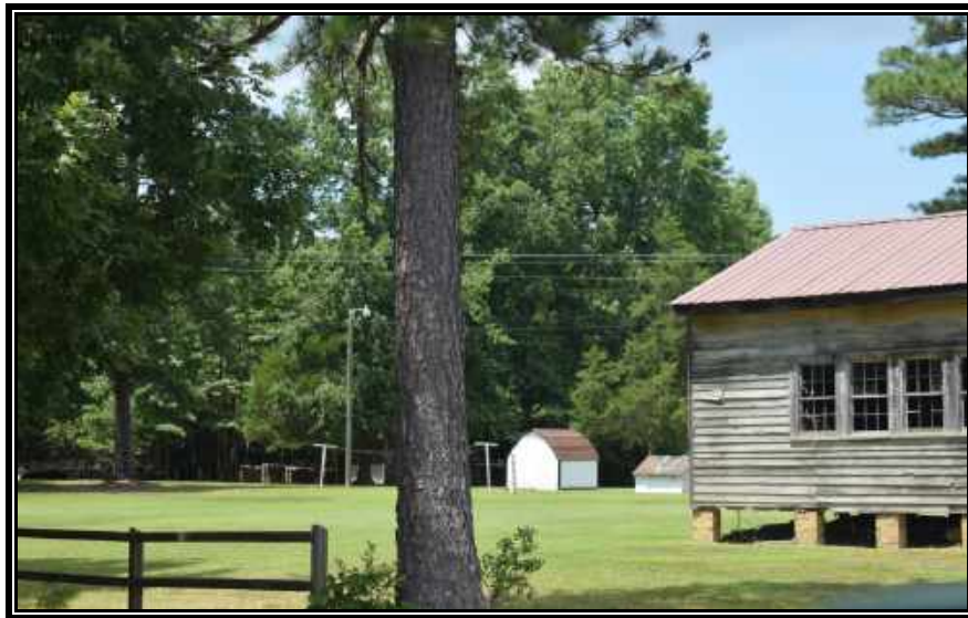
Plate 45. View of Site 090-5141, Sheds 1 and 2, and Well house, looking north.
