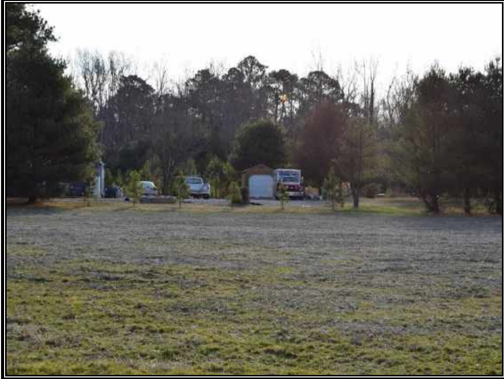
Plate 33. View of Site 090-5092, Garage, facade, looking south.
