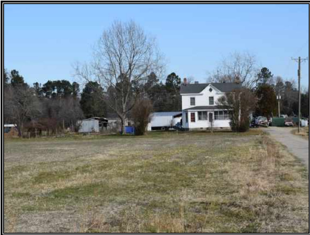
Plate 9. View Site 090-5087, House, façade, looking north.
