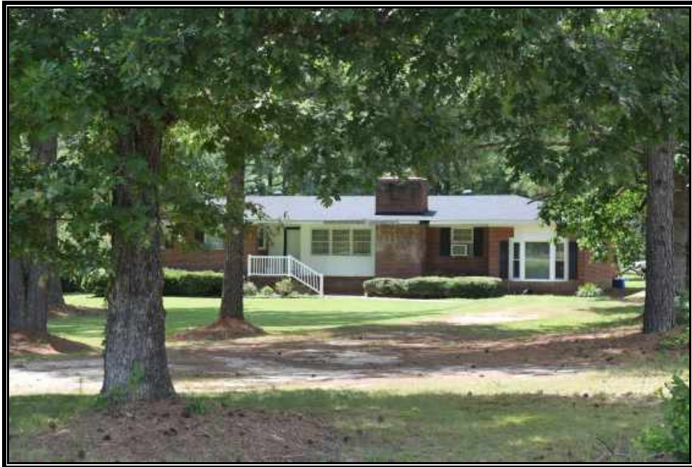
Plate 50. View of Site 090-5143, House, façade, looking west.
