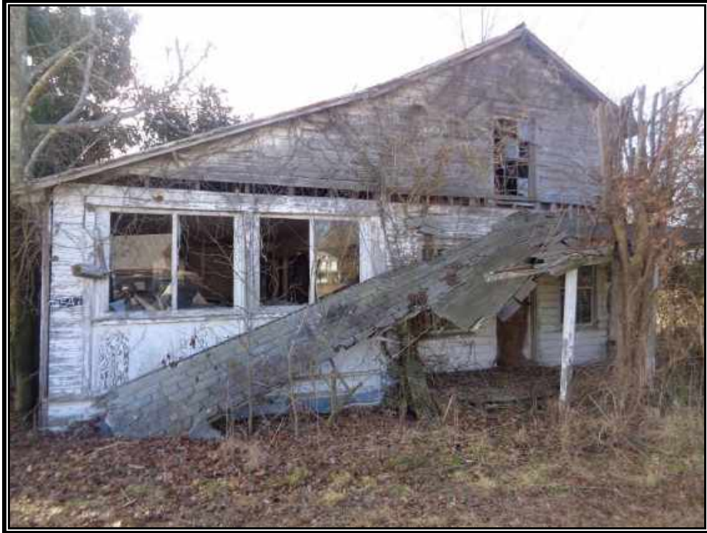
Plate 43. View Site 090-5094, Secondary dwelling, façade and addition, looking south.
