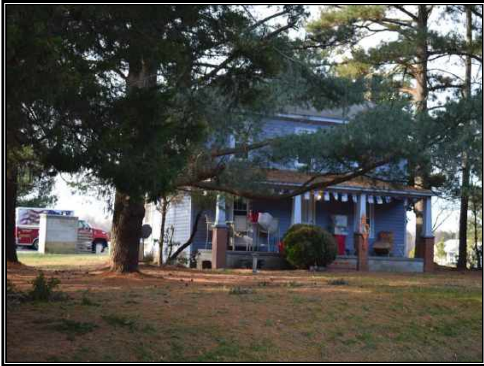
Plate 35. View of Site 090-5092, House, façade and side elevation, and Well house, looking southwest.
