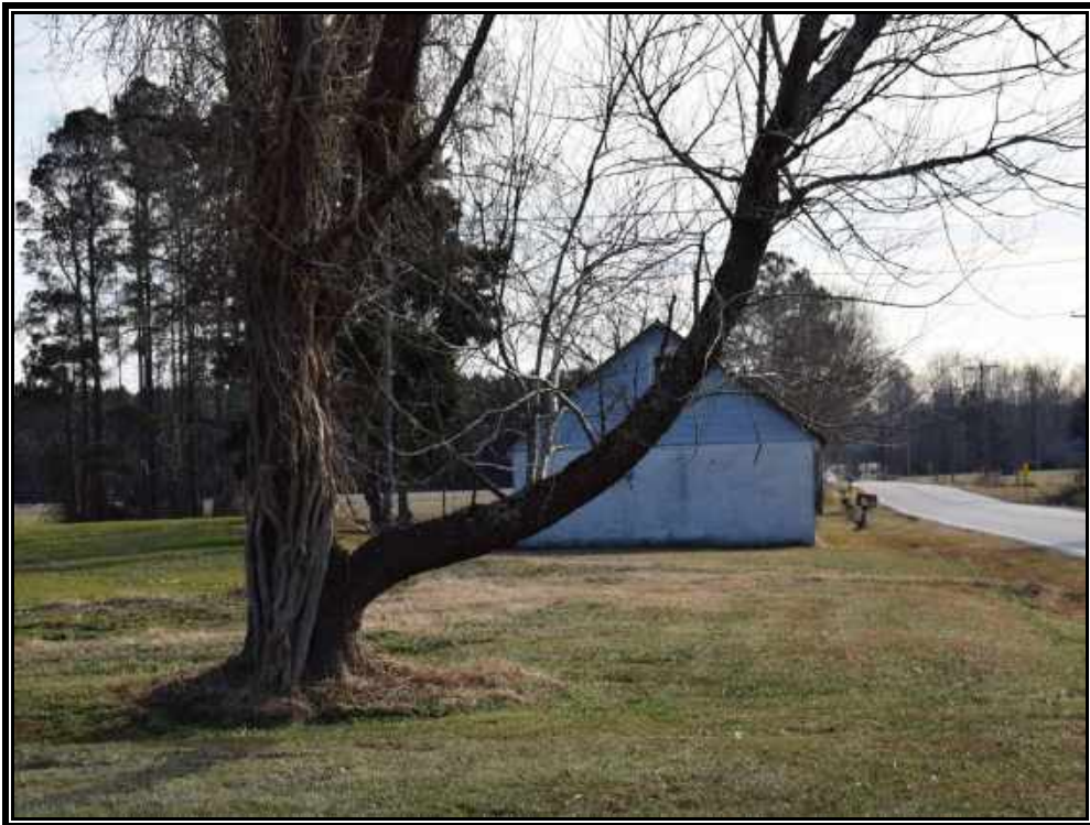
Plate 21. View of Site 090-5088, Garage, rear elevation looking east.
