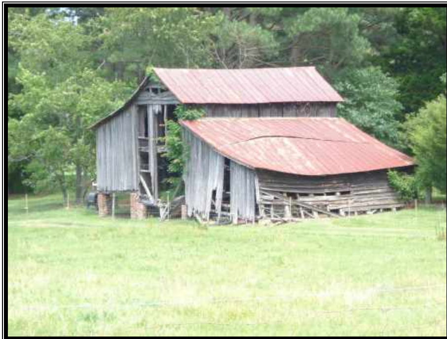
Plate 12. View of Site 090-0036, Barn, façade and additions, looking southwest.
