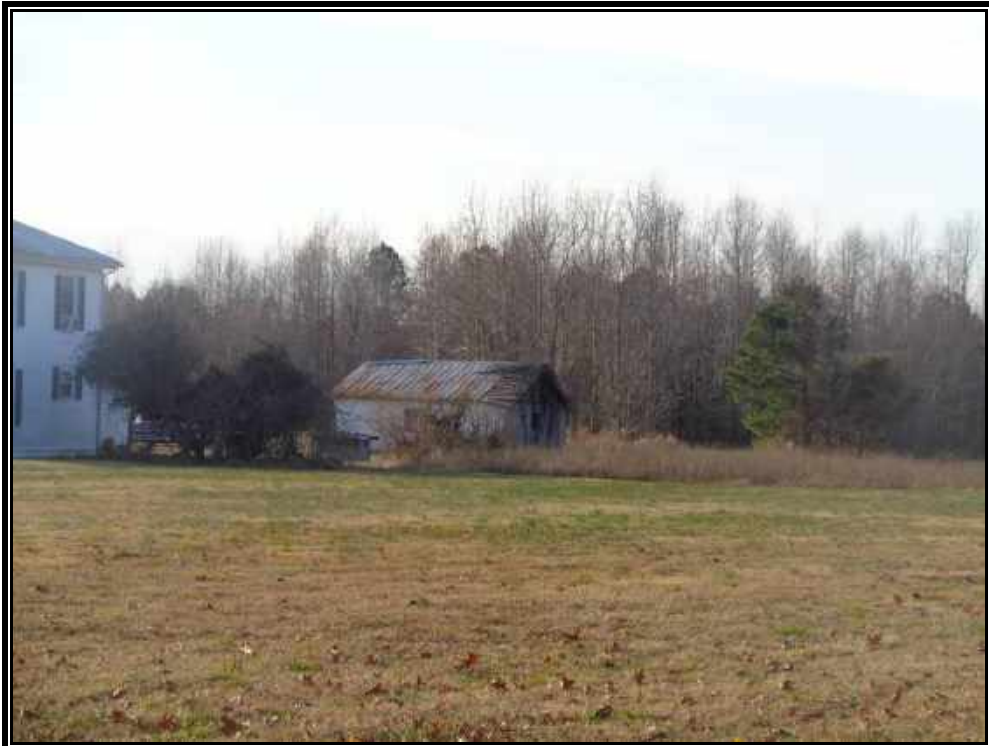
Plate 27. View of Site 090-5090, House, side elevation and addition, Barn, side elevation, and Well, looking southeast.
