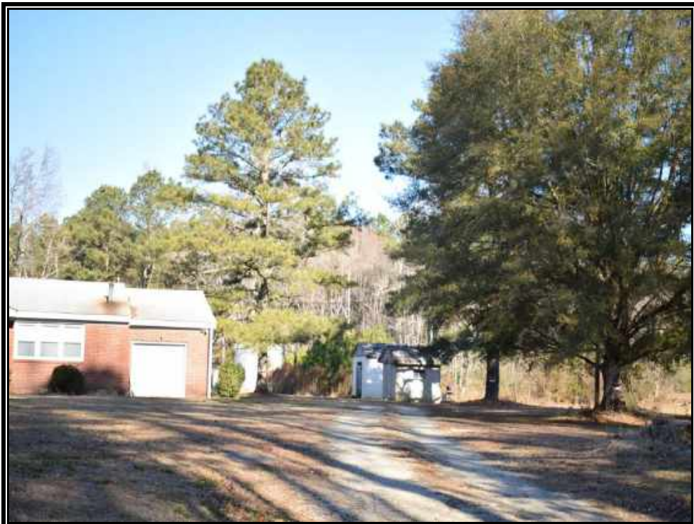
Plate 46. View of Site 090-5095, House, addition, and Sheds 1 and 2, looking north.
