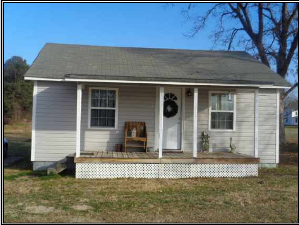
Plate 17. View Site 090-5088, House, façade, looking north.
