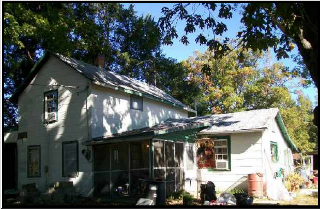
Plate 1. View of Site 090-5074, House, Façade and elevations, looking northwest.
