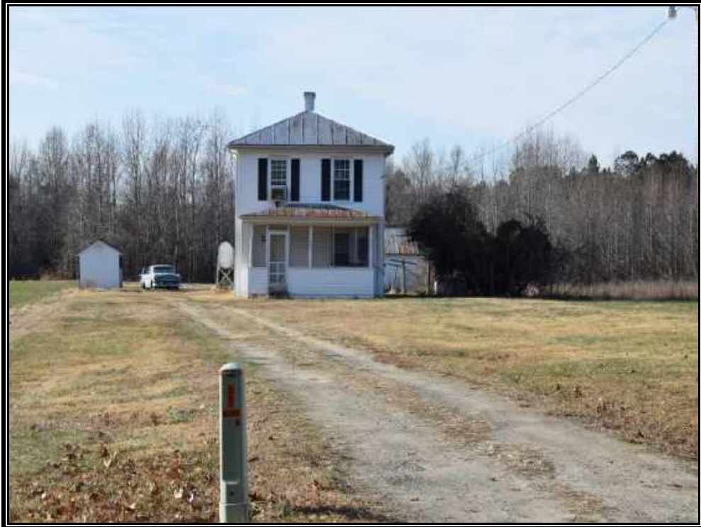
Plate 26. View of Site 090-5090, House, facade, Barn, and Shed, looking south.
