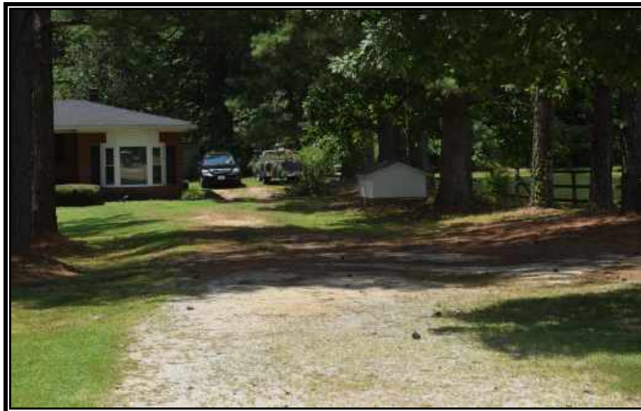
Plate 52. View of Site 090-5143, House, façade, Shed, Well house, and Well, looking west.
