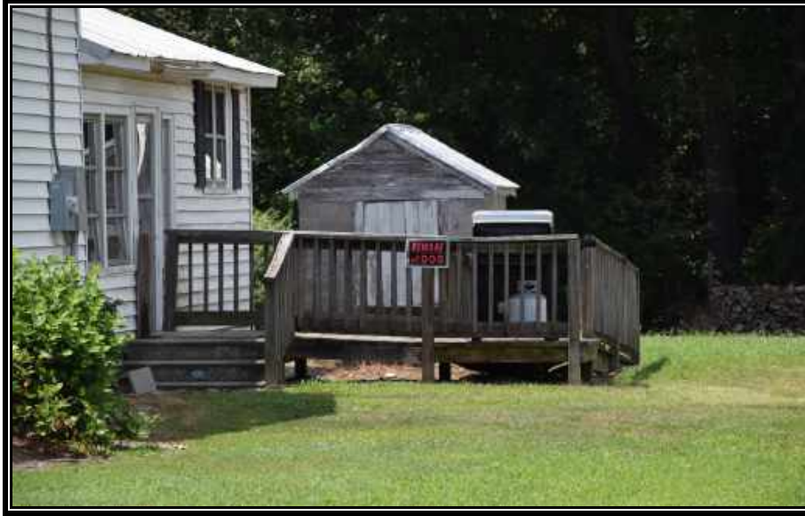
Plate 38. View of Site 090-5140, Secondary dwelling, side elevation and addition, and Shed 2, looking northwest.
