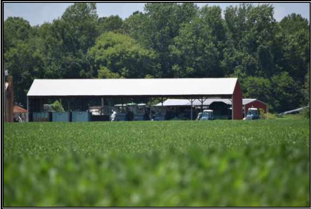
Plate 35. View of Site 090-5140, House, side elevation and addition, Pole Barns 1 and 2, and Silo, looking northwest.
