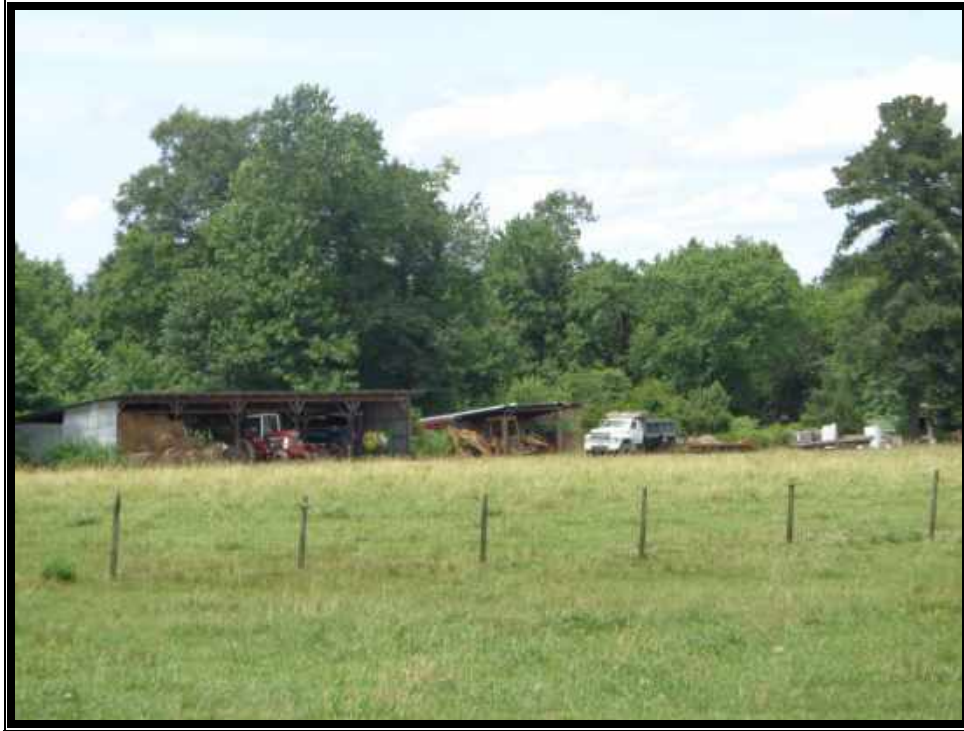
Plate 26. View of Site 090-5076, Pole Barns 1 and 2, looking northwest.
