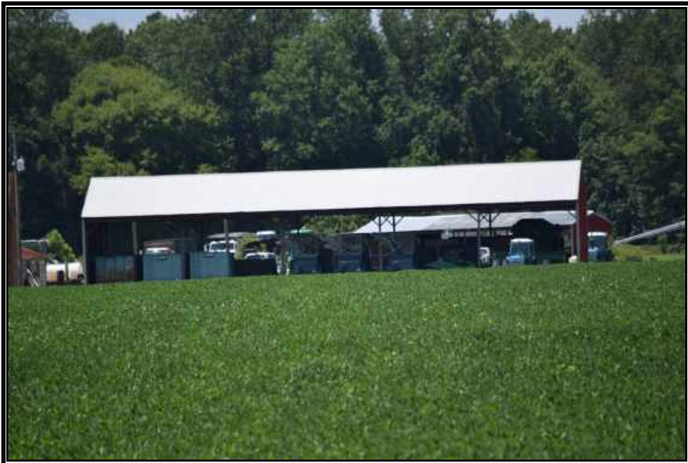
Plate 36. View of Site 090-5140, House, addition, Pole Barns 1 and 2, and Silo, looking northwest.
