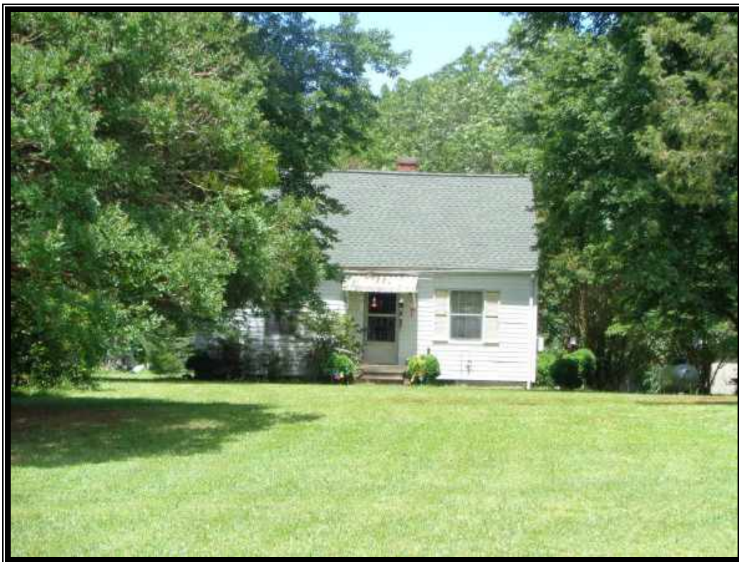
Plate 18. View of Site 090-5071, House, façade, looking north.
