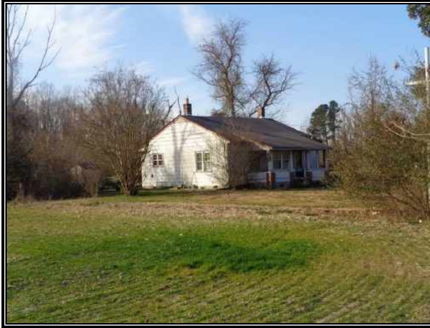
Plate 42. View of Site 090-5094, House, façade, side elevation, and addition, and Shed, looking southwest.
