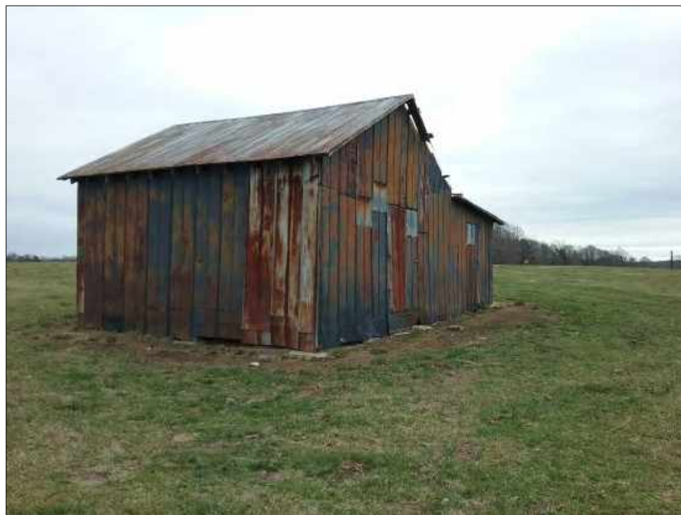
Figure 8-60: Barn associated with structural remains, facing northwest.
