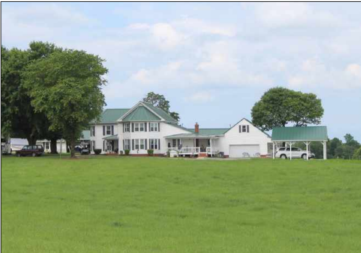
Figure 4: View 2- View of rear additions, facing west
