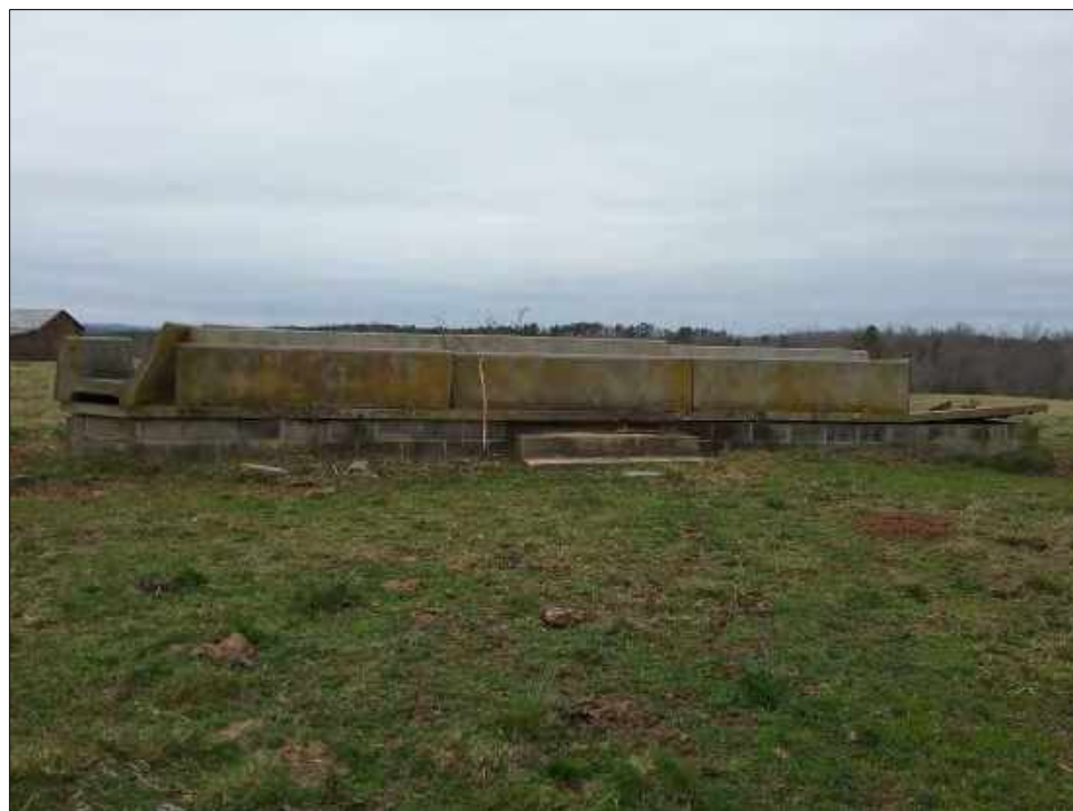
Figure 8-57: Structural remains in area C1, facing north.
