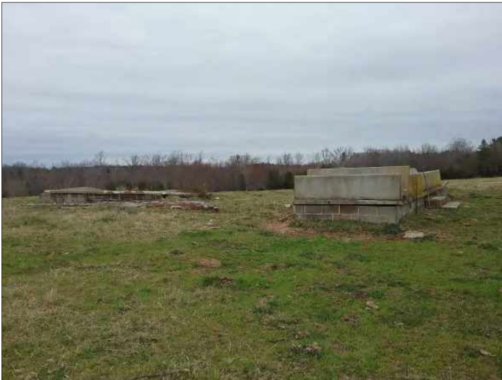
Figure 8-55: Structural remains in Area C, facing north.
