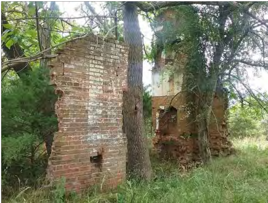
Figure 8-27: Primary resource; VDHR #034-0254, facing southwest.
