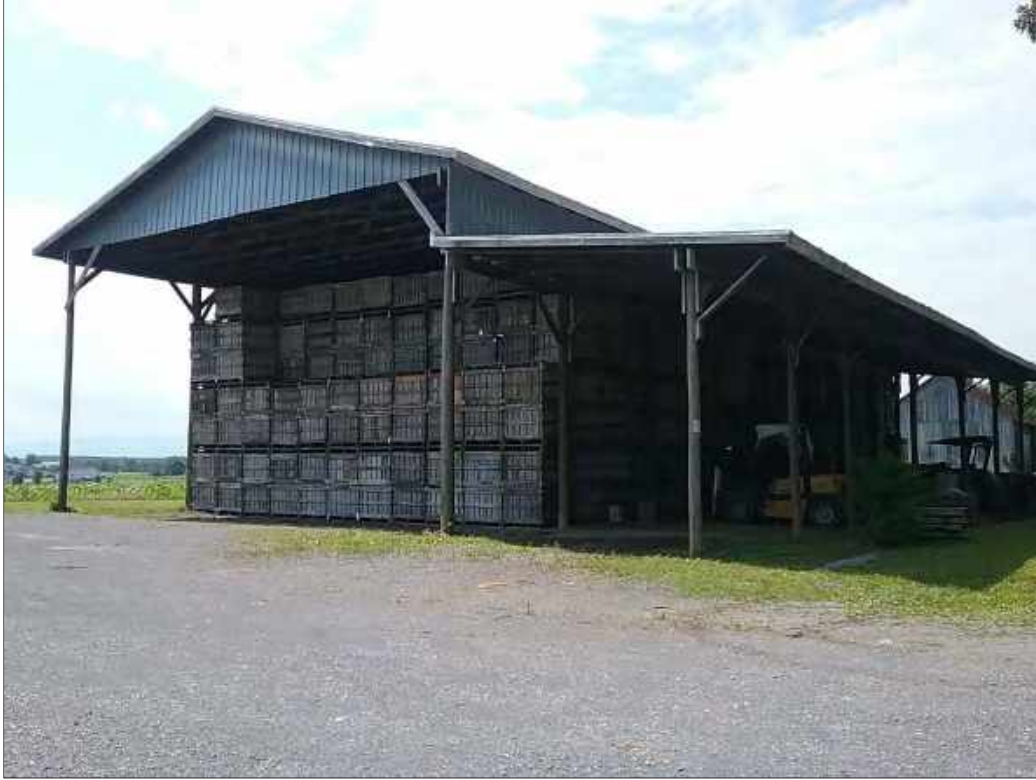
Figure 8-69: Pole barn within VDHR #034-0491, facing southeast.
