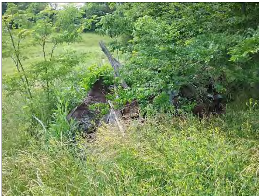
Figure 8-37: Collapsed structure, facing southwest.
