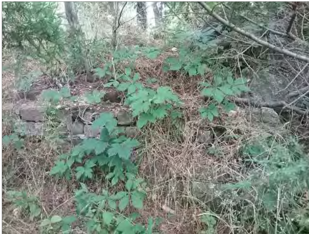
Figure 8-29: Collapsed structure, facing east.
