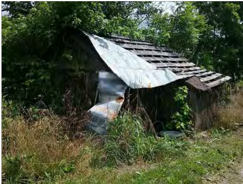
Figure 8-83: Shed in Area R, facing southeast.
