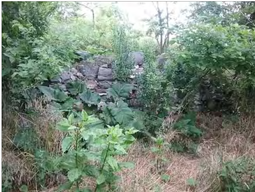
Figure 8-36: Stone foundation, facing northeast.
