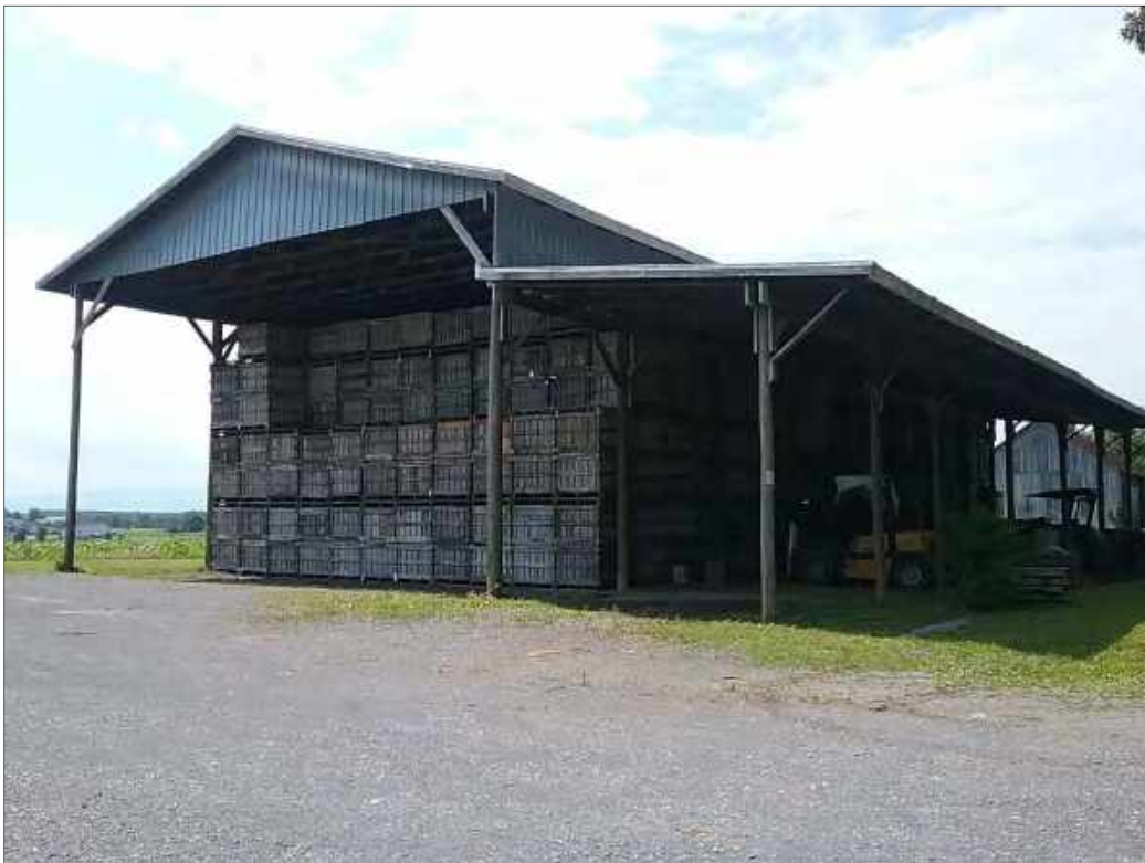
Figure 8-6: Example of pole barns for apple storage in the project area, facing southeast.
